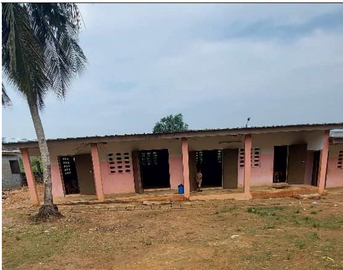
Front view of the completed building
